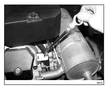
Figure 3-1 Oil Check (18 kW shown)
