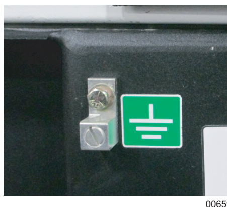
Figure 14 - Frame Ground Connection
